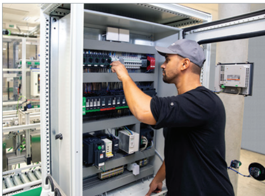
General machine control
